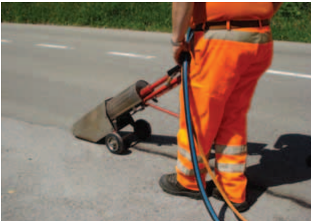
Crack repair using a Hot Dog
