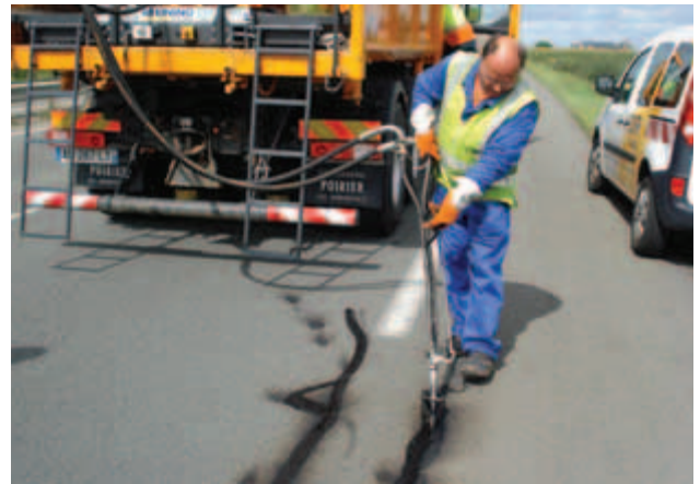
Crack repair
