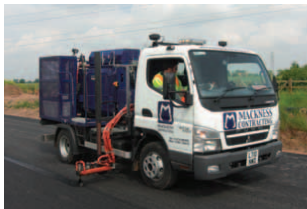
Hot bitumen slurry sealing
