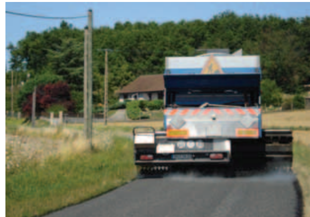
Full section slurry: Chipsealer 440CT
