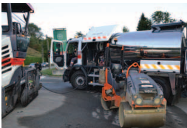
On site machinery supply
